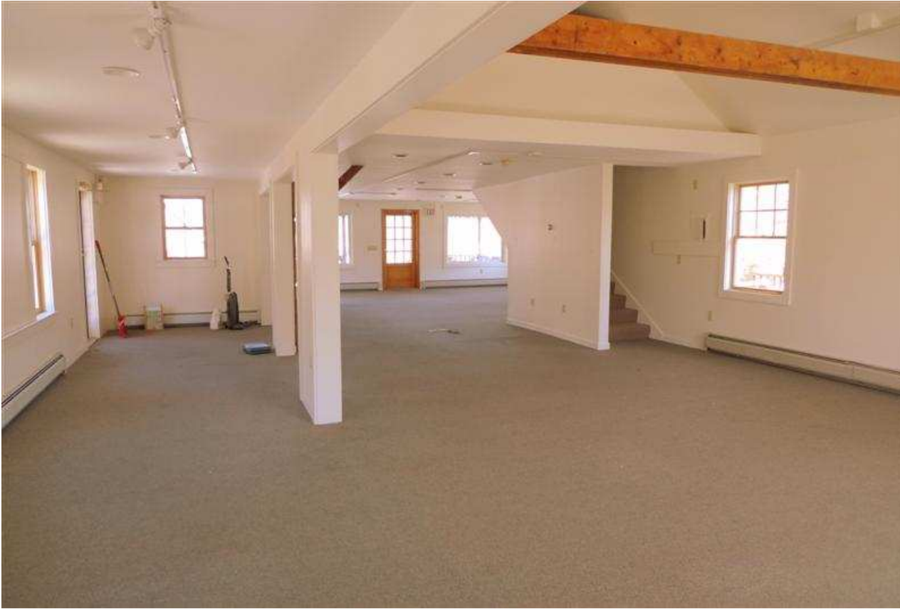
Upper Level Looking Towards Front of Building
