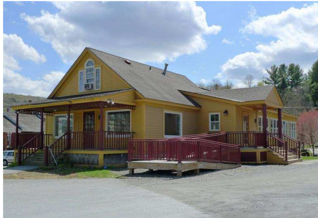
Front of Building
